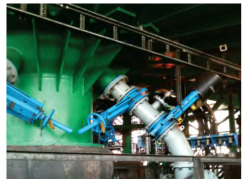
Coal Washing Plant
